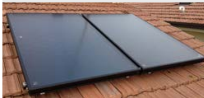
Figure 1: A picture of plate collectors (FTP)
